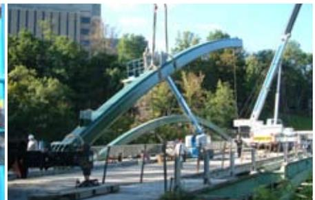
An end segment is lifted into place to attach to the bearing assembly and concrete anchor point.
