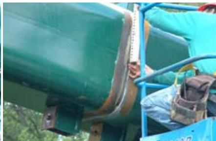
Prior to painting, areas of the arch tube are taped for the field welds.
