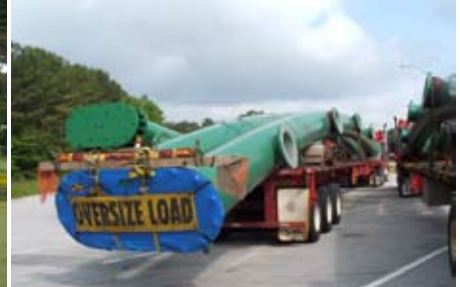
The first two arch segments are loaded on the truck.
