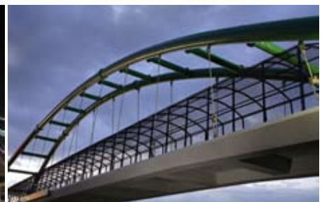
Walkways are installed on the finished bridge.
