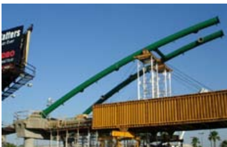
At the bridge site, the arches are erected.
