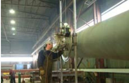
The arch gets a final inspection.
