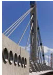
Decorative stainless steel cones fit into the concrete approach walls at each corner.
