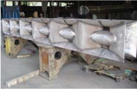
Designed for light to pass through at night, a decorative center section was fabricated and installed between the structural oval weldments in each pylon.
