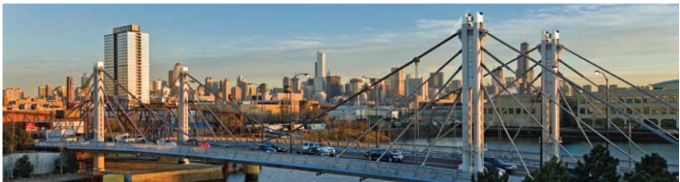
The combination suspension and cable-stay bridge was developed to meet its site parameters, which is too short for a pure suspension bridge and lacking the height clearance for a pure cable-stay design.
