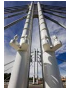
Side plates were created to hold the bridge lights.
