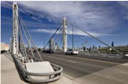
Stay cables secure the pylon towers to the deck.
